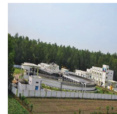
Treatment Plant, Haridwar
