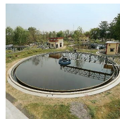
Treatment Plant, Allahabad
