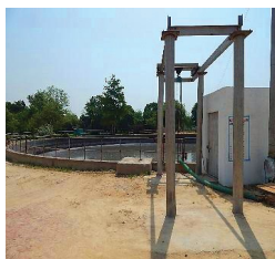
Treatment Plant, Kanpur
