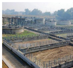
Treatment Plant, Varanasi
